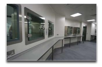
Aseptic Grade A zones were achieved through the in-house manufacture of specialist horizontal lamina airflow cabinets together with isolator provision. With licensing requirements for MHRA compliance, our in-house team supported the complete lifecycle validation programme undertaking DQ, IQ and OQ protocol preparation and execution.
